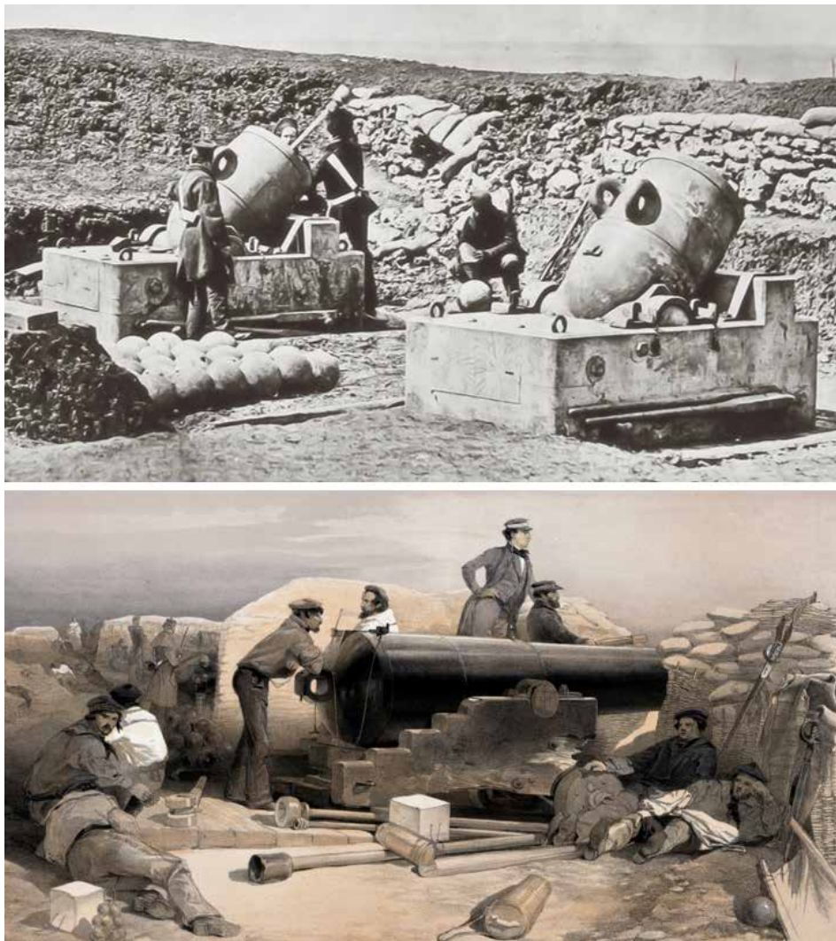
Fig. 21. The arrival of the heavy mortars and Lancaster rifled guns in the British positions at Sebastopol returned firepower superiority to the allies. A photo by Roger Fenton and a lithograph after William Simpson, respectively, 1855. Wikicommons.
